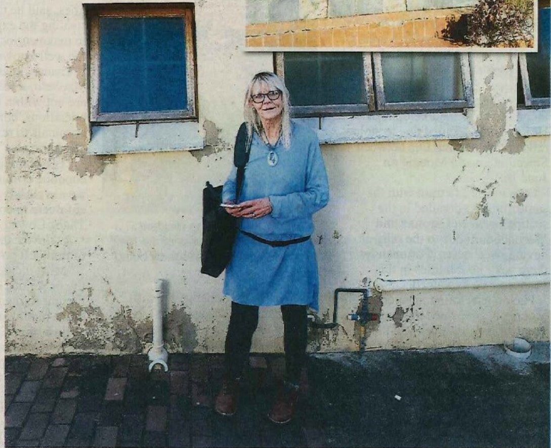
Astrid Christianson at the derelict council building. Insert: Derelict, broken floor tiles and peeling paint which greeted many visitors was cleared this week.
